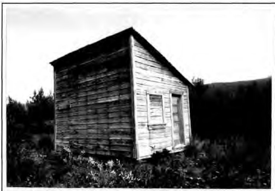
Figure 101. The Shaffrick Power Shed, 1993. The view is looking northwest.
